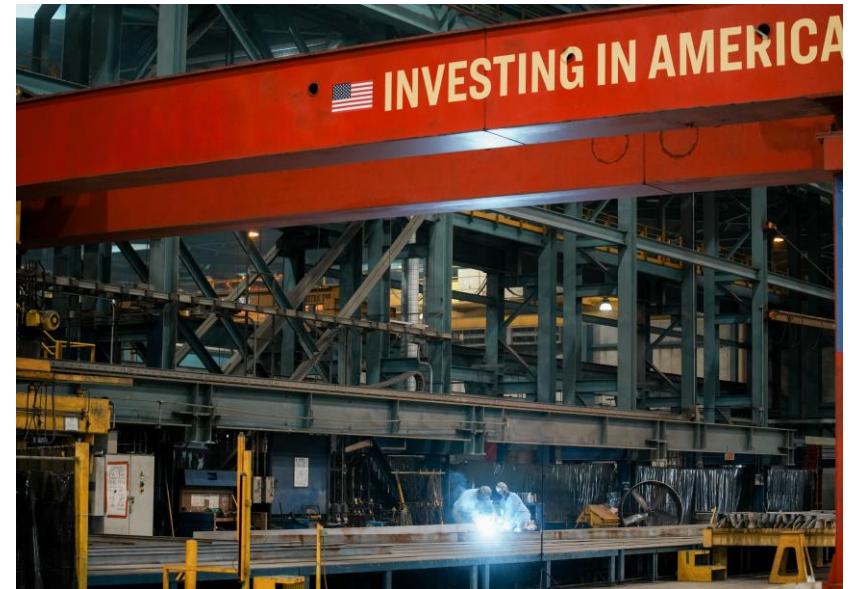
Cutting of steel at the Philly Shipyard in Pennsylvania initiates the construction of our three new “Aloha Class” vessels
