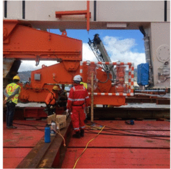
Crane is jacked up to turn the wheels.
