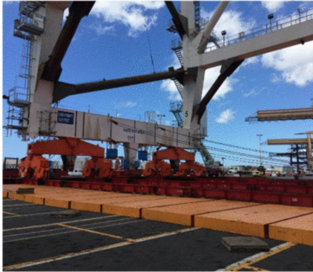
First crane off-loaded from ship to temporary rails.
