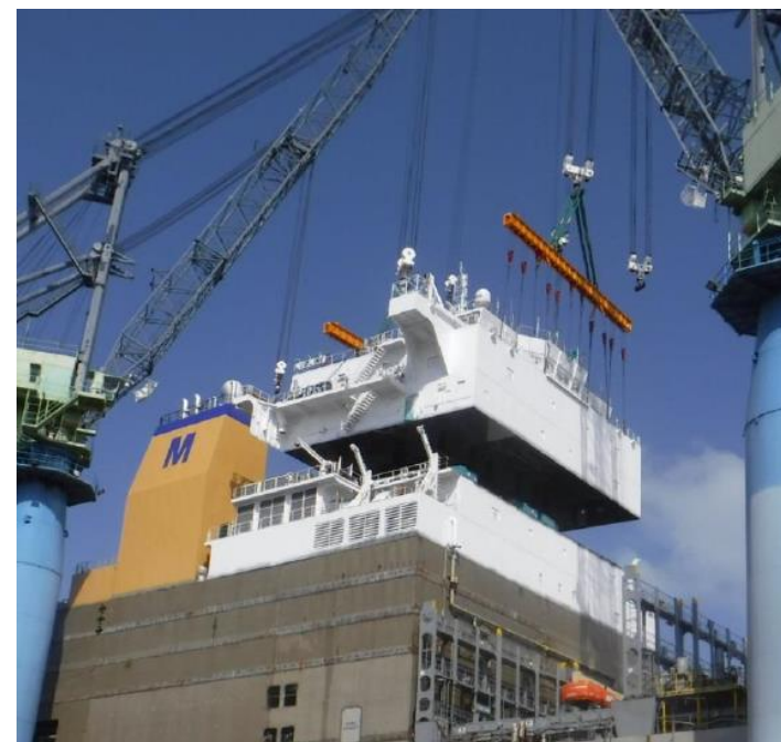
House top installation on Lurline , April 2019.
